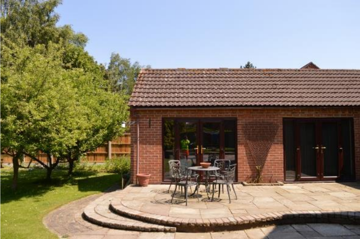
Figure 7-5: Survey viewpoint 2 – day-time looking east
